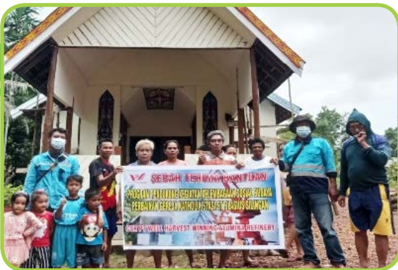
PT. Well Harvest supported the repair work of the local church
